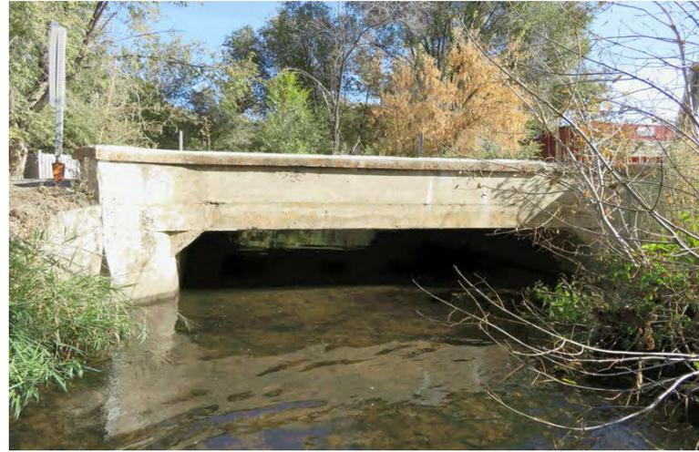
This project will replace the Rapid Creek bridge on the I-15 Business Loop between Commercial St. and Main St. The proposed bridge will address hydraulic issues that have contributed to flooding in the surrounding area. The new bridge will be wider, allowing for more pedestrian access and supporting the community's plan to improve pedestrian and cycling facilities.
